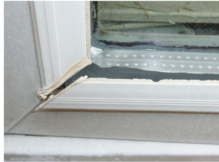
Typical failing vinyl window frame.
