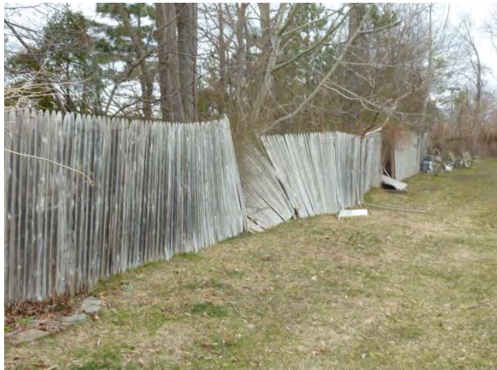
Fence along east property line should be rebuilt.
