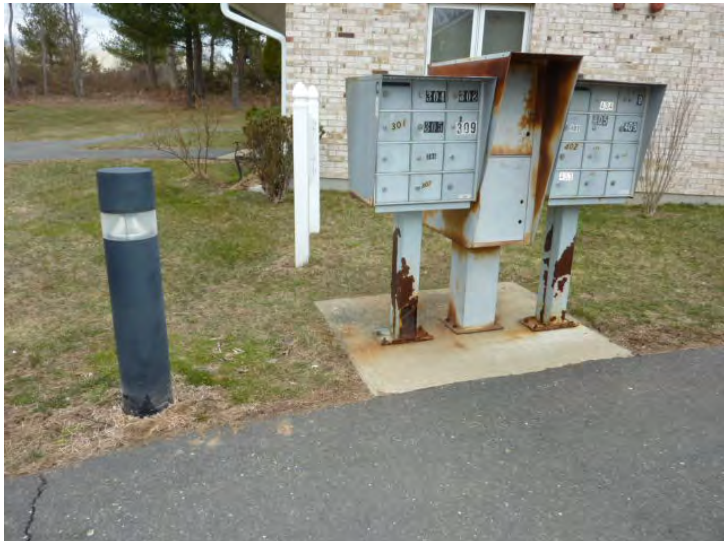
Typical rusted steel mailbox posts and hood.
