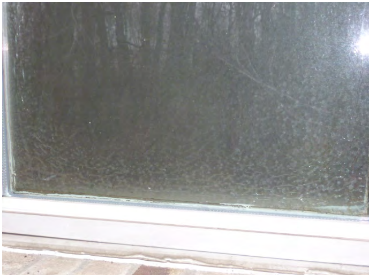
Typical condensation inside insulating glass due to failure of the perimeter glass seal.
