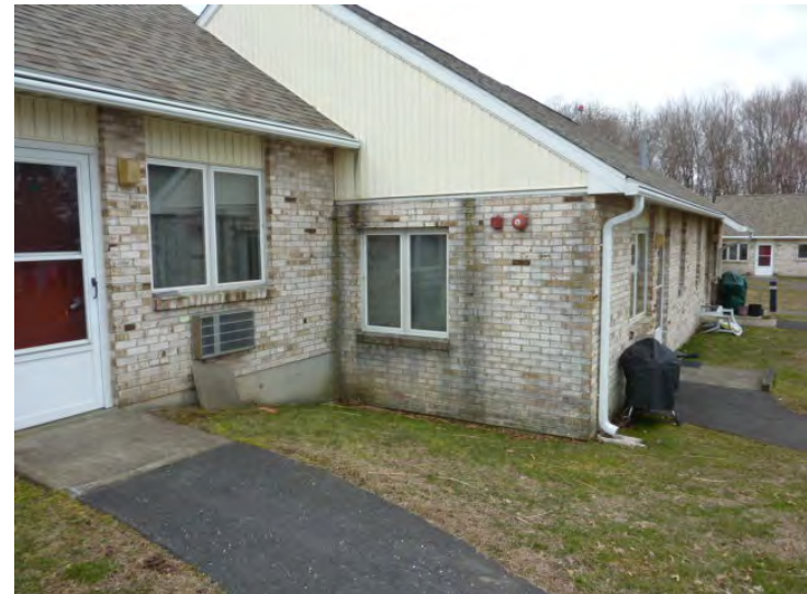
Typical staining at locations of gutters and leaders relocated in recent re-roofing project should be cleaned.
