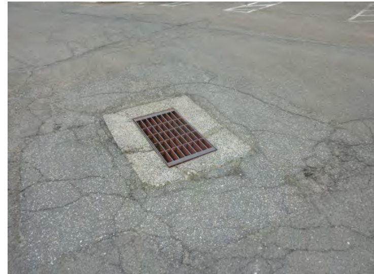
Typical sub-base failure at asphalt paving at drainage structures, drive and parking.
